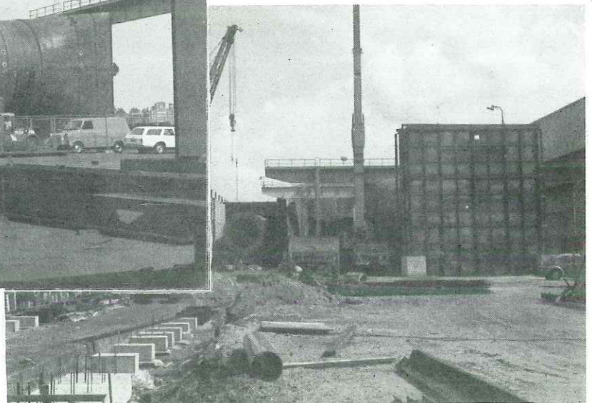
A giant 500 ton Oil Rig leg in position on dockside awaiting heat treatment.
